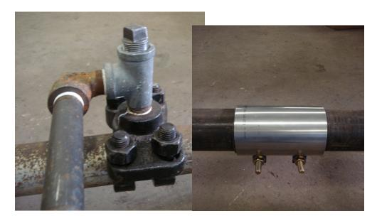
This procedure is designed for the retirement or abandonment of saddle mounted steel services that have been attached to steel gas mains operating at pressures ranging from 10 to 100 PSIG. In most installations the service tee is mounted using a mechanical "U bolt" saddle similar to those manufactured by Mueller Co. and Dresser Industries. It should be noted that this is a "No-Blow" procedure that is designed to be performed in an 18" diameter cored "Keyhole" excavation.
